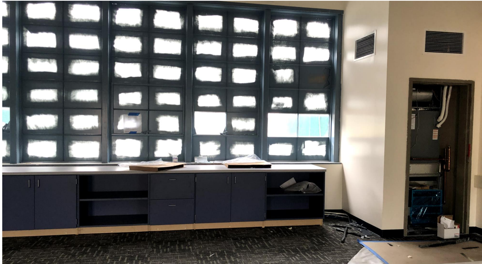
PHOTO OF ONGOING CONSTRUCTION
