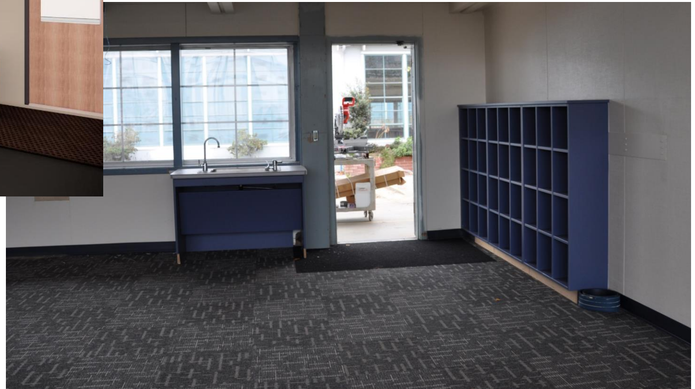
PHOTO OF ONGOING CONSTRUCTION
